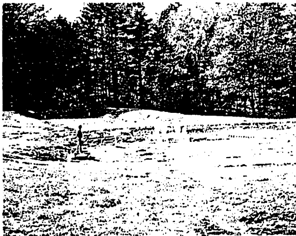
12. After excavation, grading, and compaction, a newly-constructed wetland is ready for planting.
